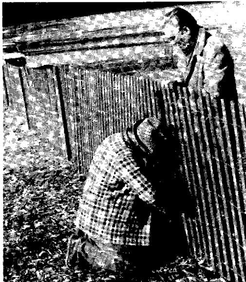
Figure 1. Ed Rothe and Roger Brown installing snow fence to protect the Preservation Program's hybrid azalea collection at USDA's Plant Introduction Station in Glenn Dale, Maryland.
