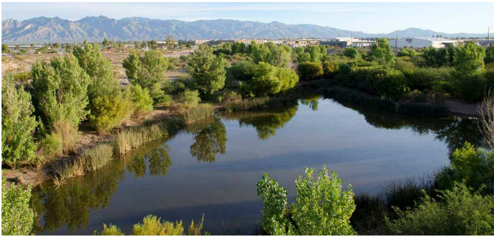
The Kino Ecosystem Restoration Project near Tucson Boulevard and Ajo Way may be southern Arizona's largest stormwater harvesting facility. Runoff sustains wetland and native riparian vegetation but is also piped outside the basin for use on the Kino Sports Park and roadway medians. Credit: Brian Powell, Pima County.
