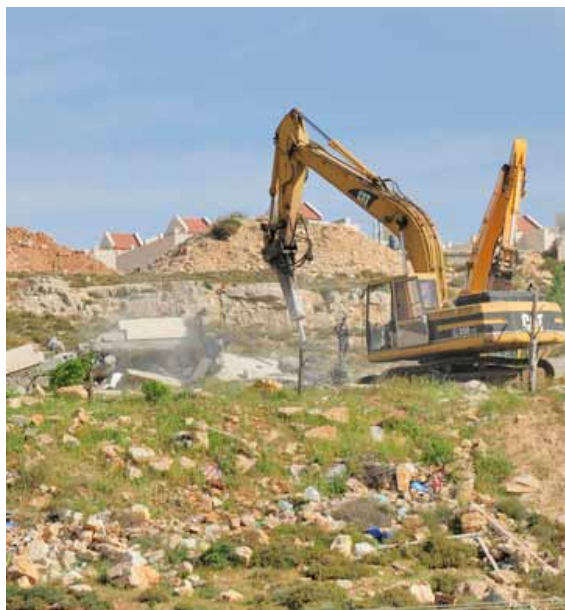
Demolition in Beit Hanina in East Jerusalem, 2011. (© Virginia Paradinis)
