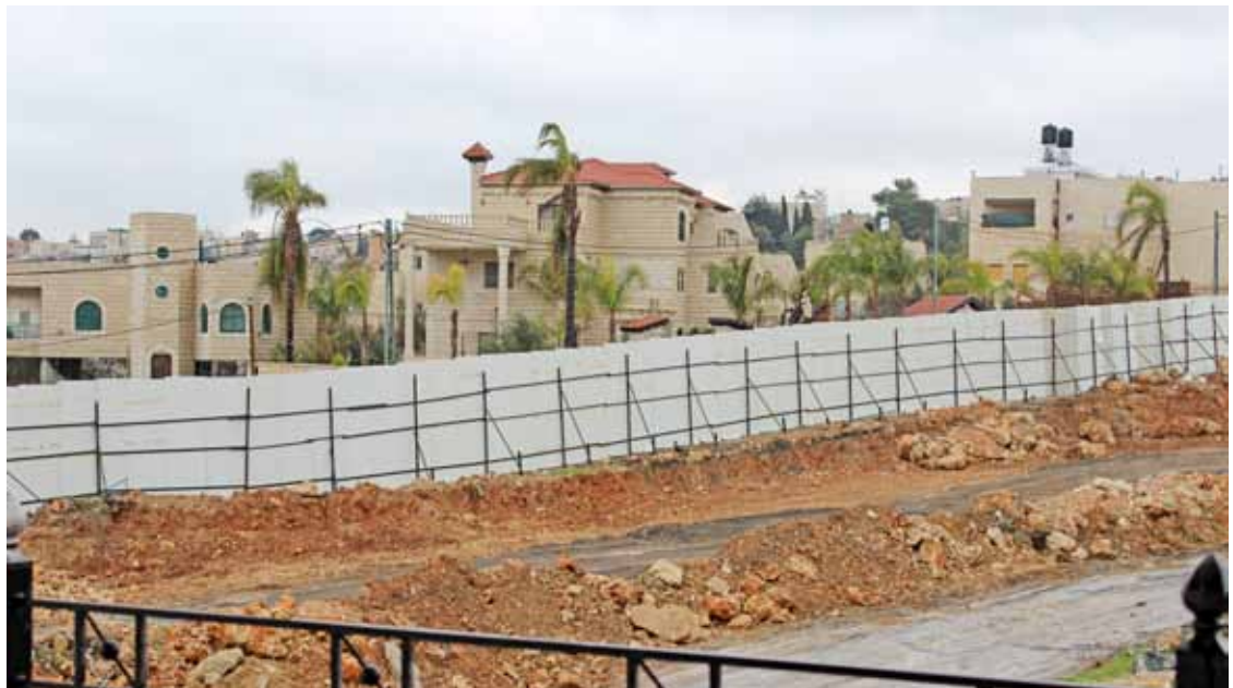
Construction of Road Number 50 (Begin Highway) in Beit Safafa, February 2013. (© BADIL).
