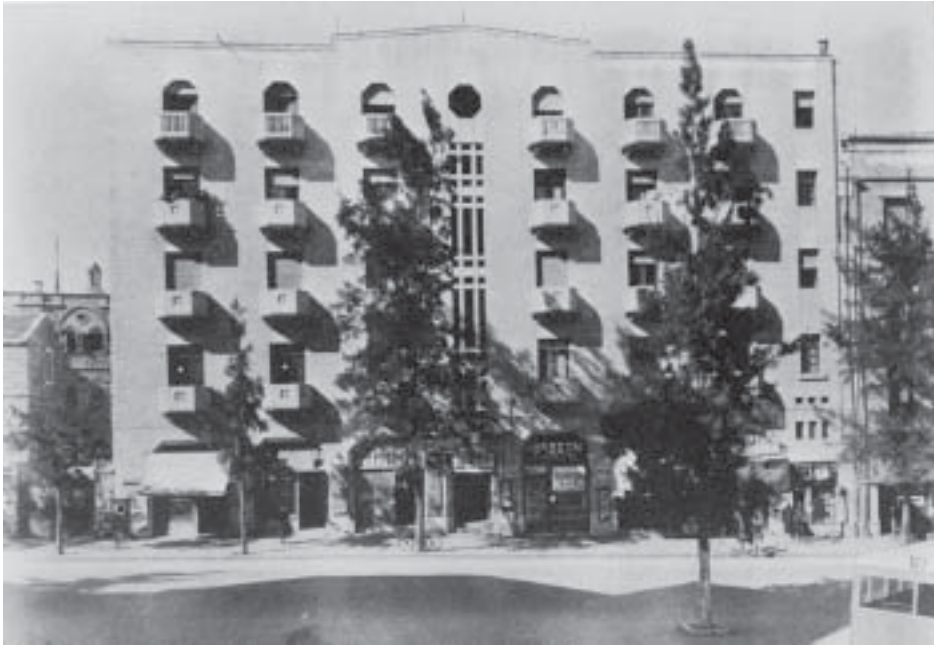
Tannous building, King George Street, early 1940s. Photographer unknown, reprinted from Before their Diaspora.
