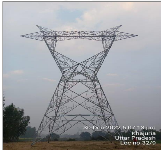
765kV & 400kV D/C LILO lines under TBCB
