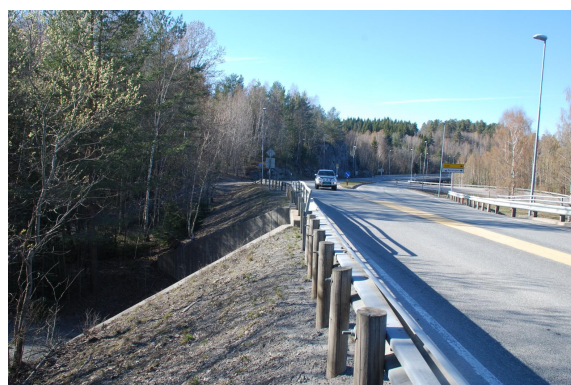
Figur 4-8 Kulvert under fv. 353
