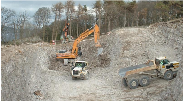
Figure 38 Example of loading at the face
