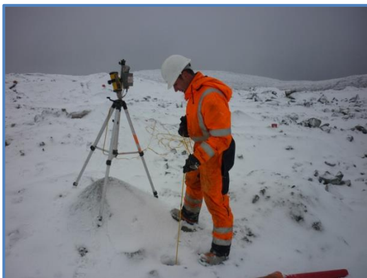
Figure 26 – Surveyor using electronic probe to survey holes
