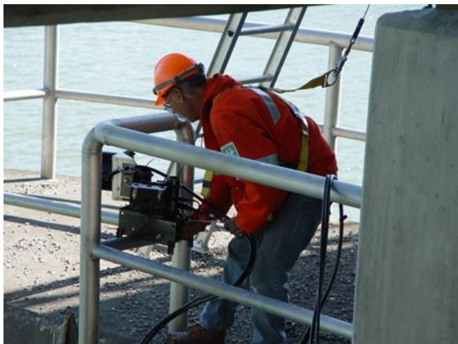
Installation of hydro acoustic transducer at the dam.
