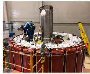
A crew member touches up paint on a rotor at BR2.
