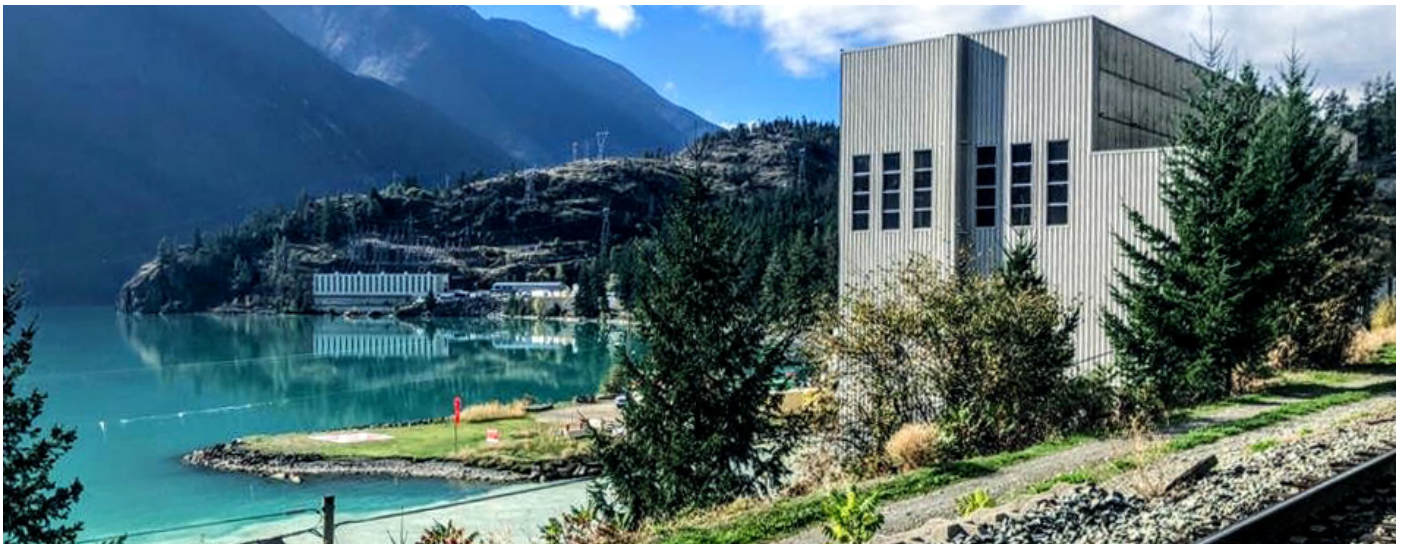
The powerhouses at Bridge River
