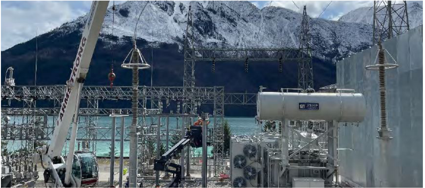
Crews install steel components in late March as part of the Transformer 3 Replacement Project at Bridge River 1. The project is expected to be completed this summer.
