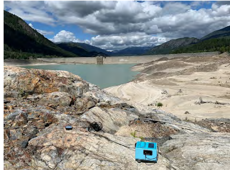
Above: Measuring ground vibrations around the dam.
