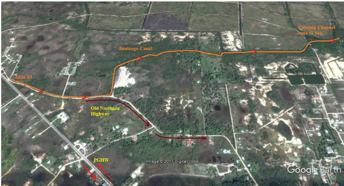
Figure 6.17: Drainage Canal at Mile 13 PGH.
