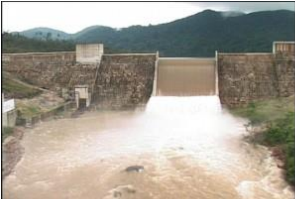
Figure 6.32: Chalillo dam spilling after period of heavy rainfall.
