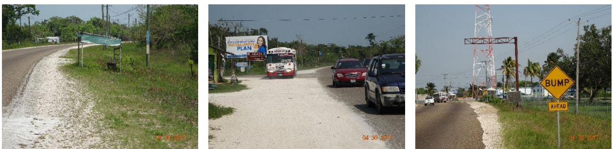
Figure 2.12: (Left) Unauthorized covered bus shed too near the edge of the pavement, creating visibility problem; (Center) public transport using Old Northern Highway access road as bus stop this in the absence of a designated bus lay-bys; (Right) missing directional signs at major intersection of the Burrell Boom road and the PGH.
