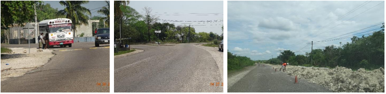
Figure 2.13: (Left) Public transport using the carriageway as a bus stop for the embarkation of passengers; (Center) lack of traffic signs and the need to maintain solar powered caution flashing light; and (Right) no safety signs were noted on this major potable water main installation works along the PGH.
