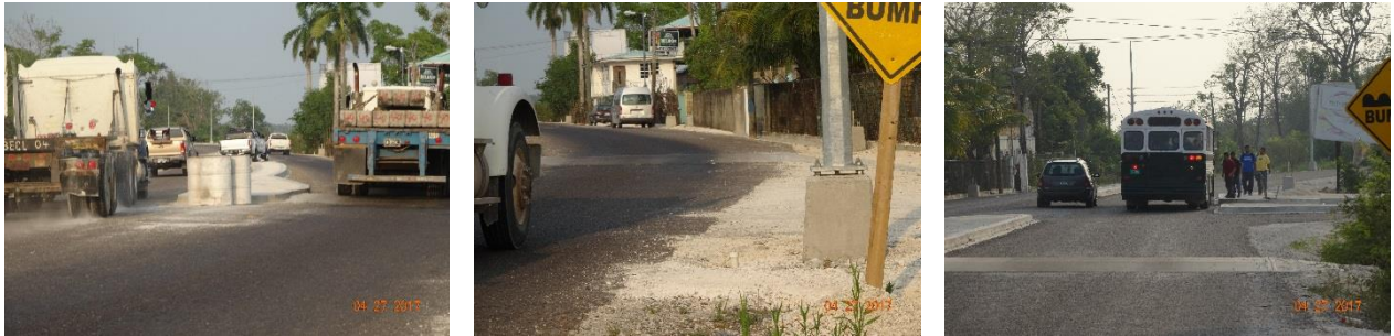
Figure 2.10: Road safety concerns at Vista Del Mar Junction mile 8.5 with the PGH. (Left) Illegal overtaking at junction; (Center) utilities are near the pavement edge and (Right) bus stops lay-bys are required.
