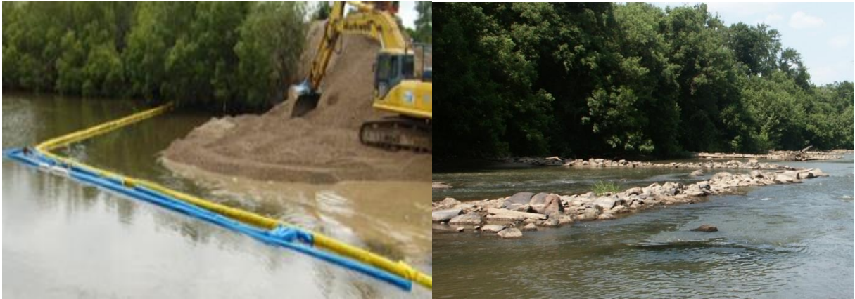
Figure 6.13: Wing Dams (L) Silt Screen (R) Natural rocks.
