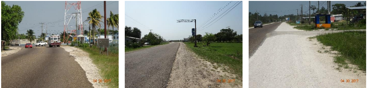
Figure 2.9: Pavement surface along Section 2. (Left) Pavement near the Burrell Boom junction surface in fair conditions, no paved shoulders no line marking and broken pavement edge; (Center) Pavement in fair condition, shoulder drop in dire need of replenishment, signs are outstanding at the old Northern highway junction; (Right) Pavement surface in fair conditions with recently completed shoulder replenishment works which since is not sealed creates a dust pollution problem.
