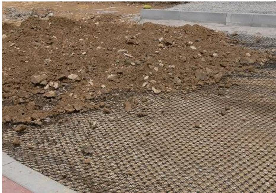
Figure 6.11: Geomats used for ground stabilization.
