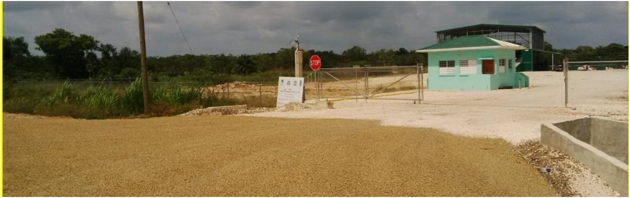
Figure 6.20: Burrell Boom [Solid Waste] Transfer Station. (Source SWAMA, Belize 2017.)
