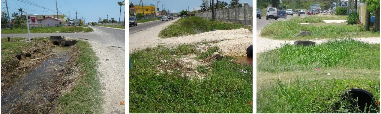
Figure 2.1 Longitudinal side drains Ladyville Village.
