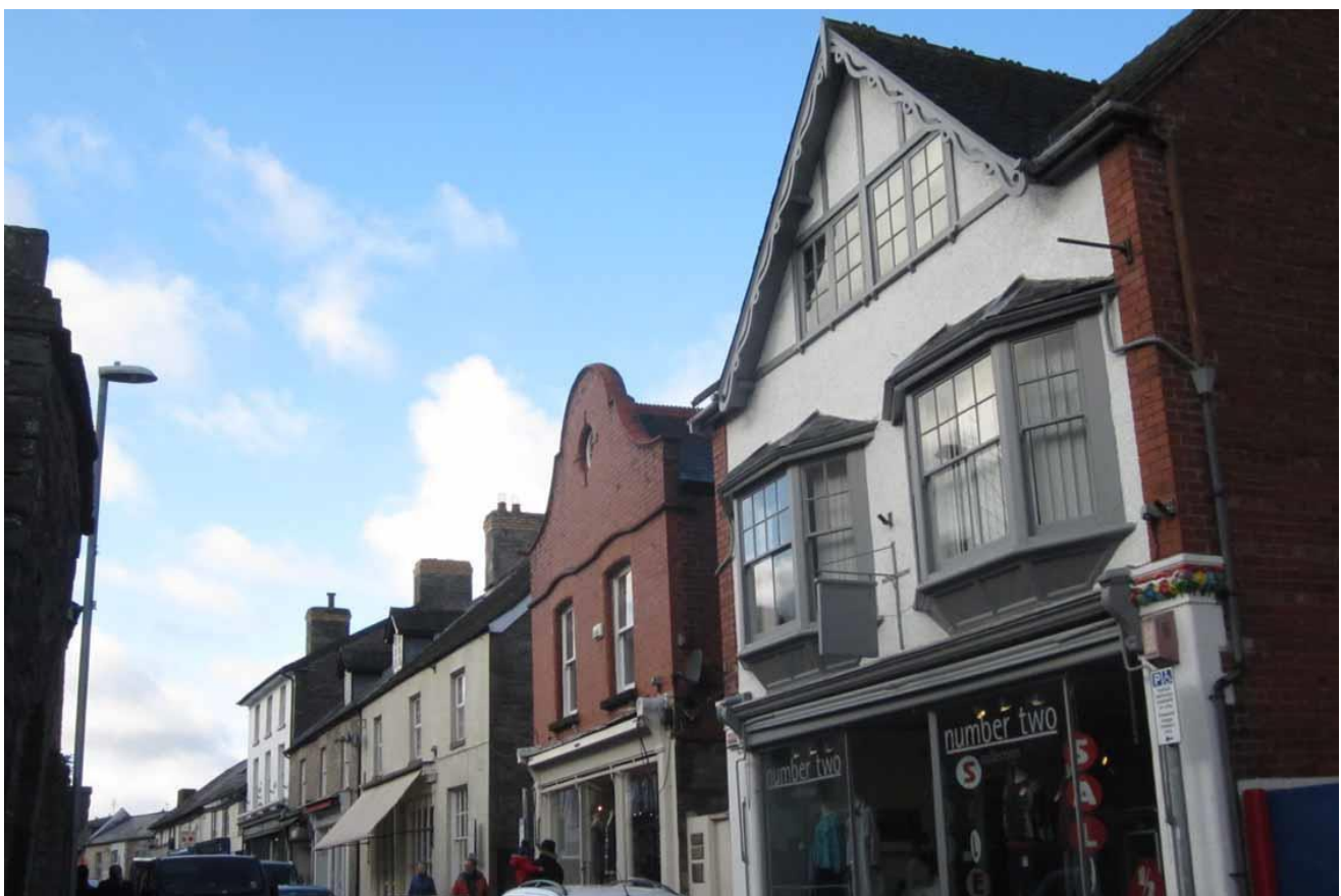
The variety of elevational treatment within Castle Street
