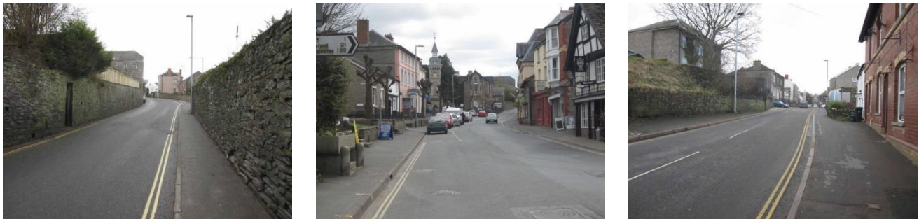
There are significant changes in character along the length of the street with the narrow enclosure of boundary walls of Belmont Road (left), the wide, civic space of Broad Street (centre) and a softer character integrated with the landscape in Newport Street (right)
