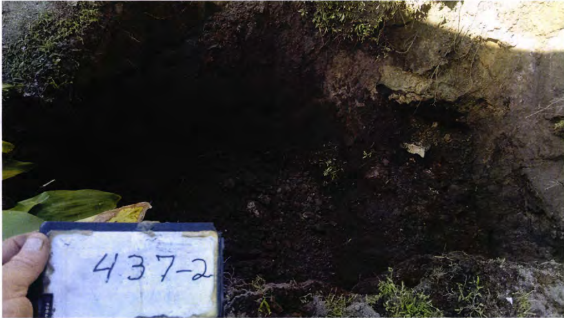
Picture 3: UST 437Elderberry-2 excavation.
