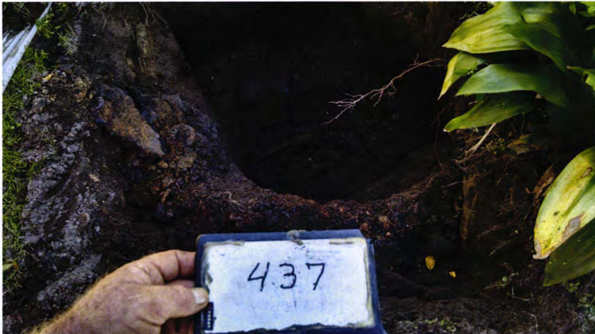
Picture 2: UST 437Elderberry-1 excavation.
