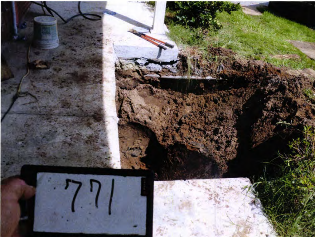
Picture 2: UST 771Althea excavation.
