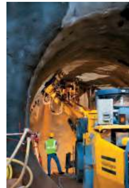
^^ | London Underground modernization
