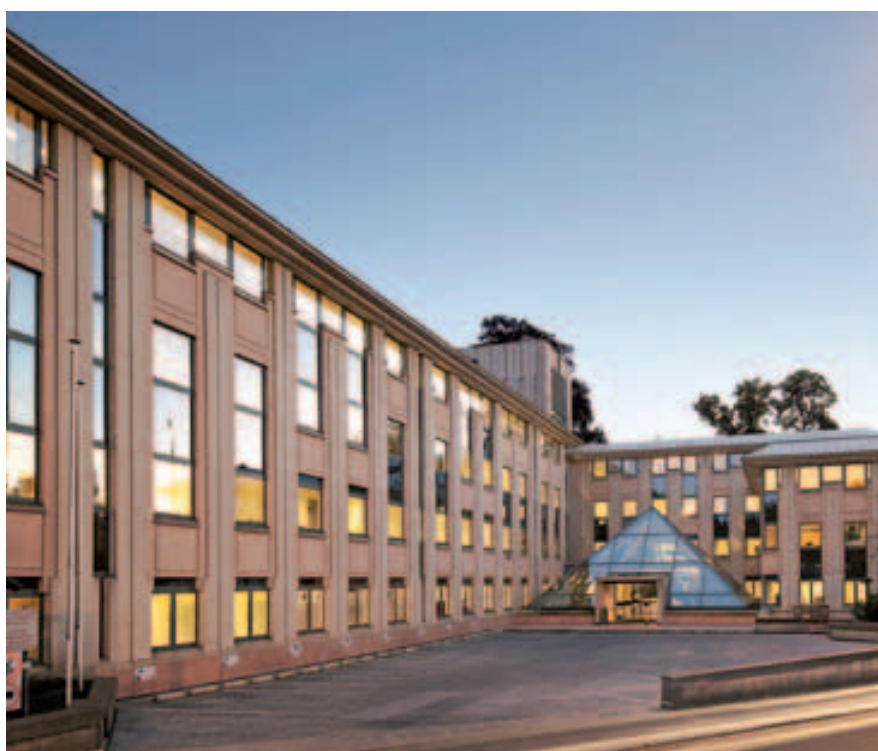
Goemaere, Brussels decentralised
