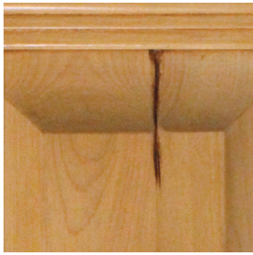
#9 - GOUGES (ADD 10%) Large, deep area where the wood is removed (deeper and wider than "cracks").
