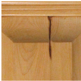
#9 - GOUGES (ADD 10%) Large, deep area where the wood is removed (deeper and wider than "cracks").
