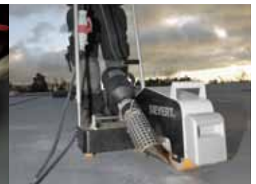
TW 5000 hot-air welding
