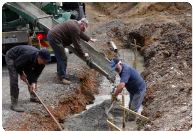
Footings for the Chinese Pavilion
