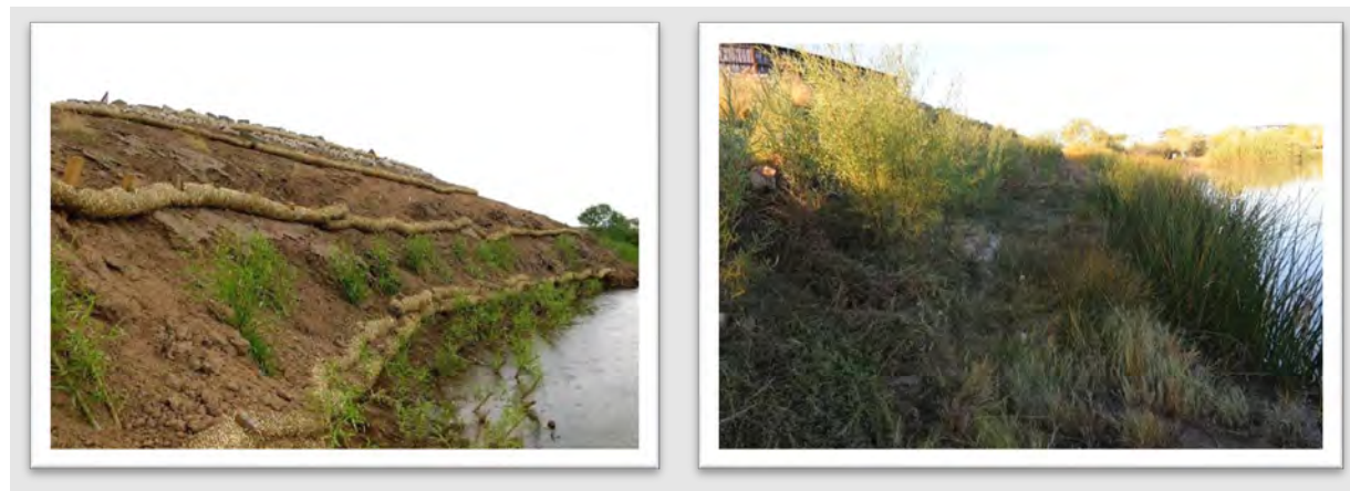
Figure 10-2. Bundles of fast-growing plants planted along the streambank can provide erosion control when steep banks cannot be re-graded. Left: grass bundles installed along a steep bank with willow bundles planted in between to stabilize and capture soils on the bankline. Right: The same bankline one year later. Photos courtesy of Fred Phillips Consulting.
