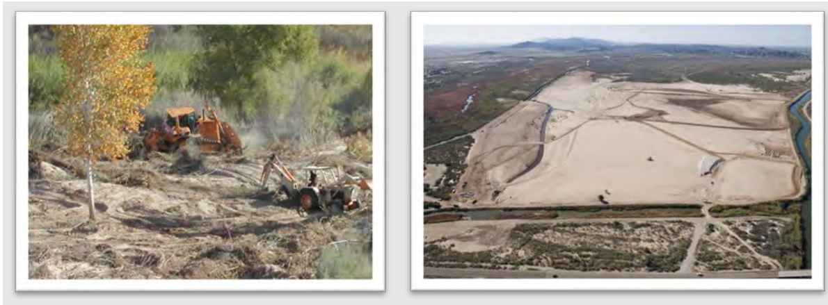
Figure 9-1. Examples of mechanical treatments. Left. Tractors grubbing root systems for large tamarisk stands. Right. A site cleared of invasive tamarisk using mechanical treatments. Photos courtesy of Fred Phillips Consulting, LLC.
