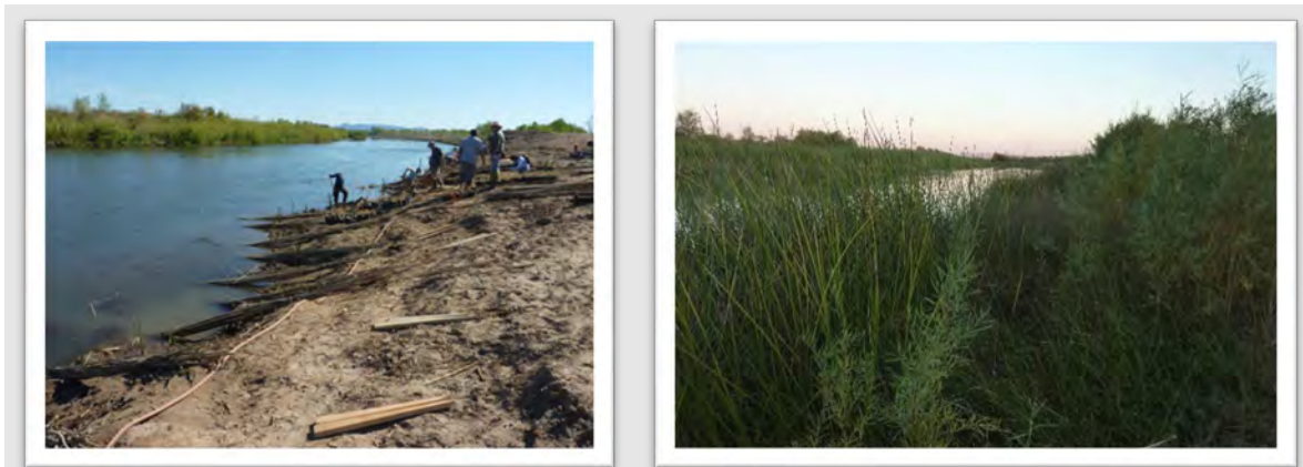
Figure 10-1. Harvested willow poles are planted along a bankline to provide additional erosion protection. Left: Work crews prep the bundles of willow poles after they have soaked in the Colorado River. Right: the same location one year after planting. Photos courtesy of Fred Phillips Consulting.
