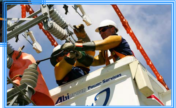
High Voltage Arm Replacement Melbourne
