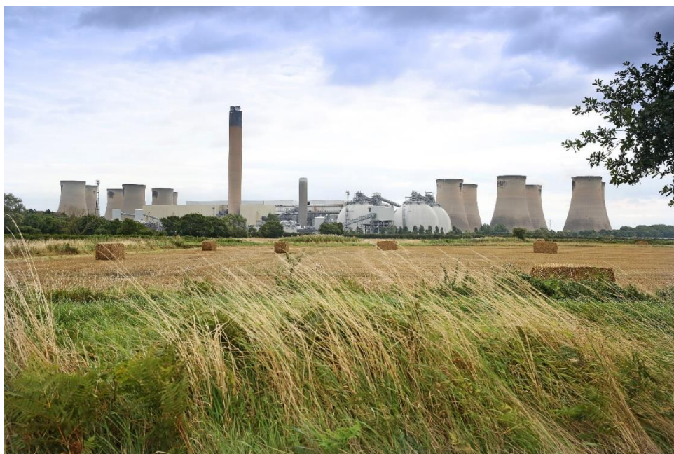
Figure 33: The Drax power station in Selby, UK; the biomass storage domes are visible (Source: Drax Group )
