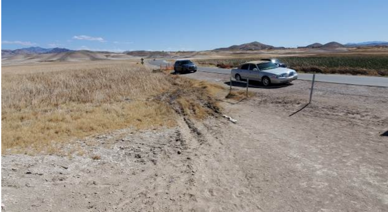
Figure 6: users have driven around the fence at the parking area and into the marsh. March 21, 2021.
