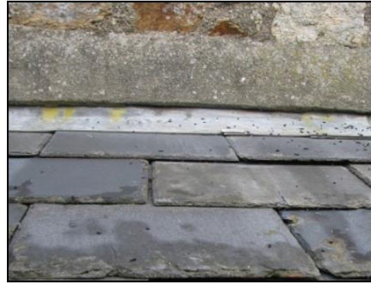
Close up, note the yellow staining and droppings on the lead flashing
