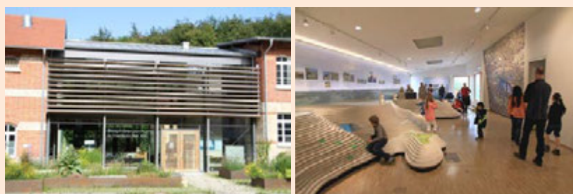
Figure 48: Biosphere Centre (left) and the nature conservation centre Schopflocher Alb (right), as example for a local information centre (BR Administration).
