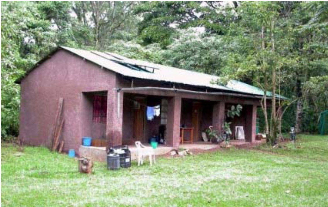
Fig. 1. Newly constructed BIOTA laboratories at KWS campsite Buyangu, Kakamega Forest, Kenya.
