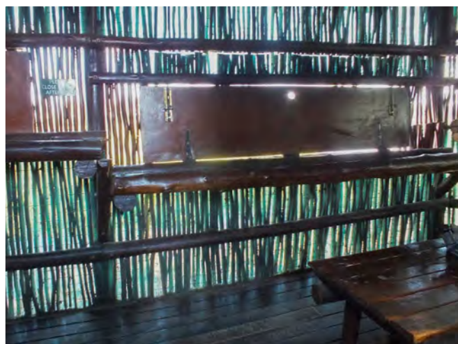
RIGHT And some of the viewing slots have been lowered so that children, wheelchair users and other height compromised people can enjoy the views from Maloutswa © Chris Patton.
