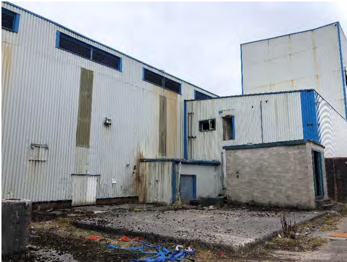
Photograph 4: Openings in wall on northern side of building A.
