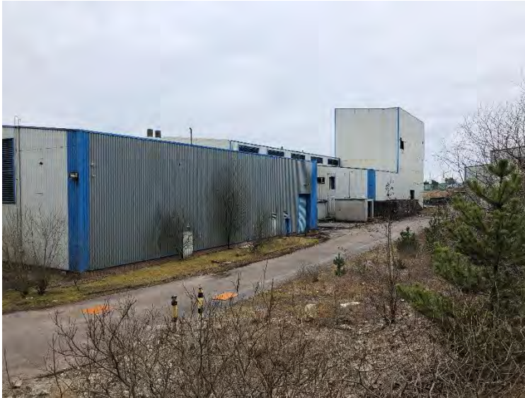
Photograph 1: View of the northern aspect of Building A.
