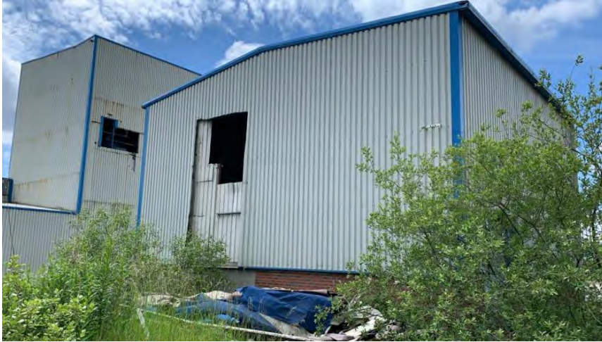
Photograph 5: large opening on eastern side of Building B.
