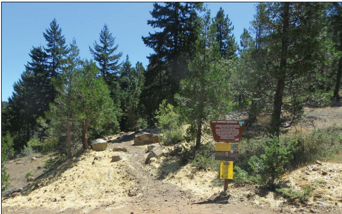
Road-to-trail conversion – Pilot Rock Trailhead
