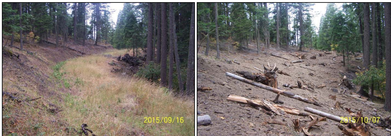
Before/After photos – road removal in the SMW
