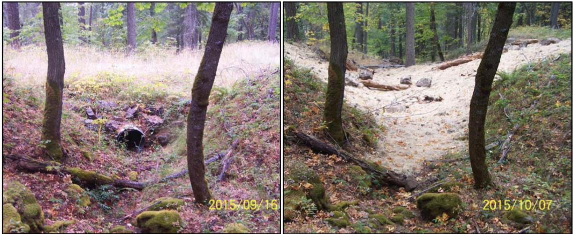
Culvert removal and restoration
