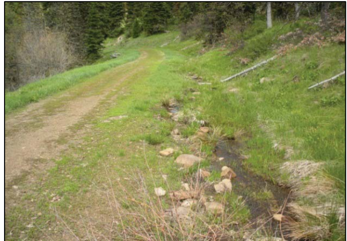
Example of altered hydrology on legacy road in SMW
