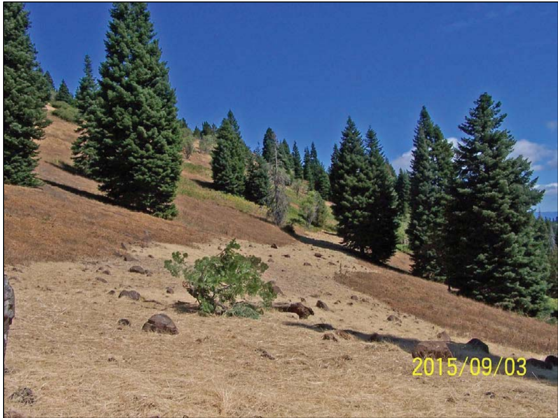
Road removal on Soda Mountain
