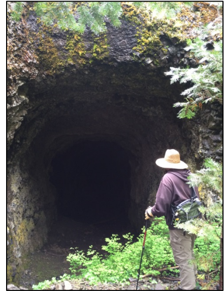
Buck Rock Tunnel
