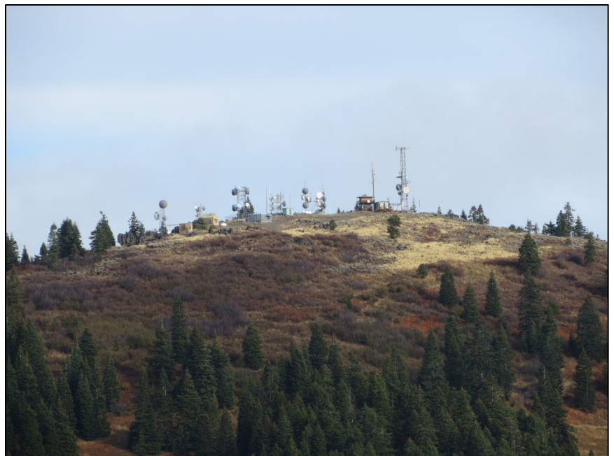
Telecommunication towers on Soda Mountain
