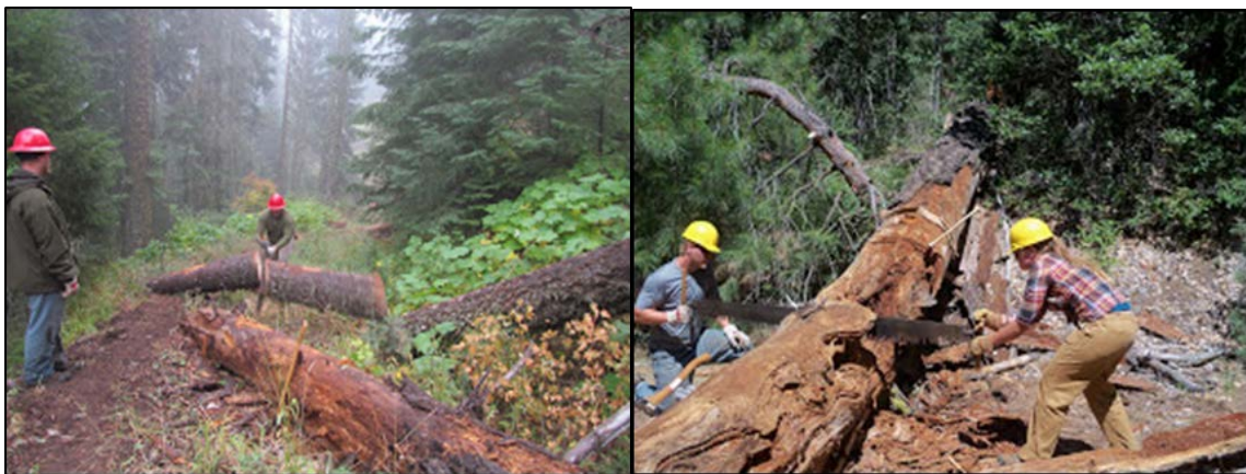
Volunteers clearing the Pacific Crest National Scenic Trail
