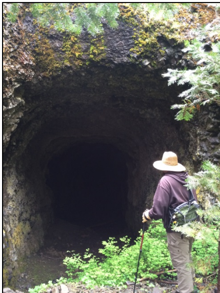
Buck Tunnel – potential trail site
