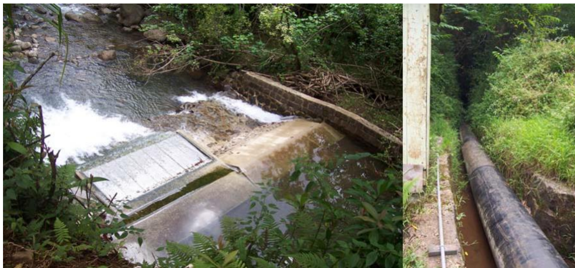
Figure 1.7 Punalu’u Stream Diversion and Piped Ditch
