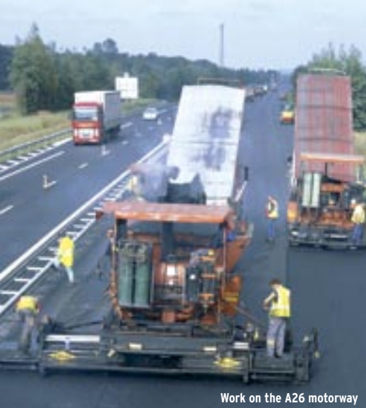
Work on the A26 motorway
