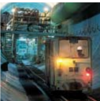
Sydney metro: a 6-km tunnel delivered for the 2000 Olympics.
