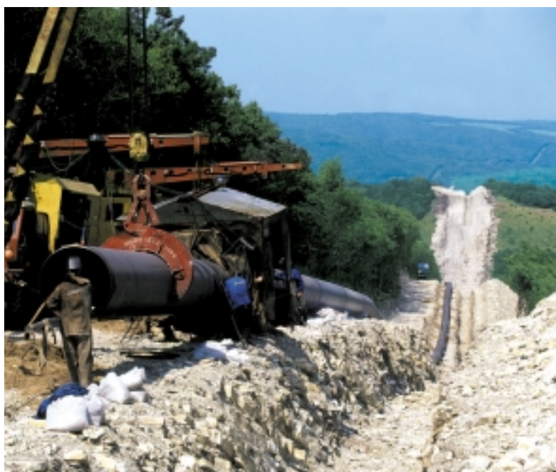
Laying pipelines in Russia.
