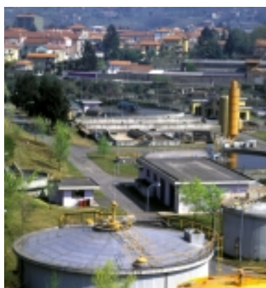
Verbania wastewater treatment plant in Italy.
