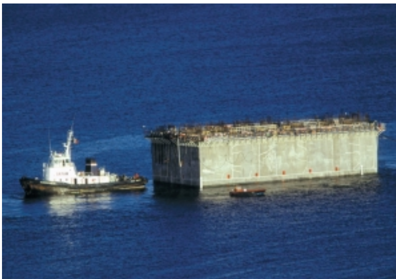
Transporting pre-fabricated caissons for the Monaco breakwater.
