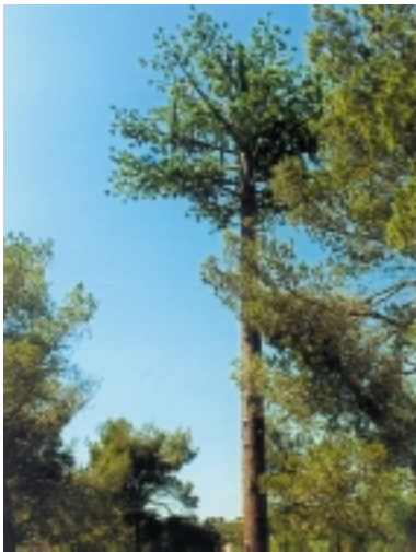
Bouygues Telecom conceals its aerials with tree camouflage, for example.
