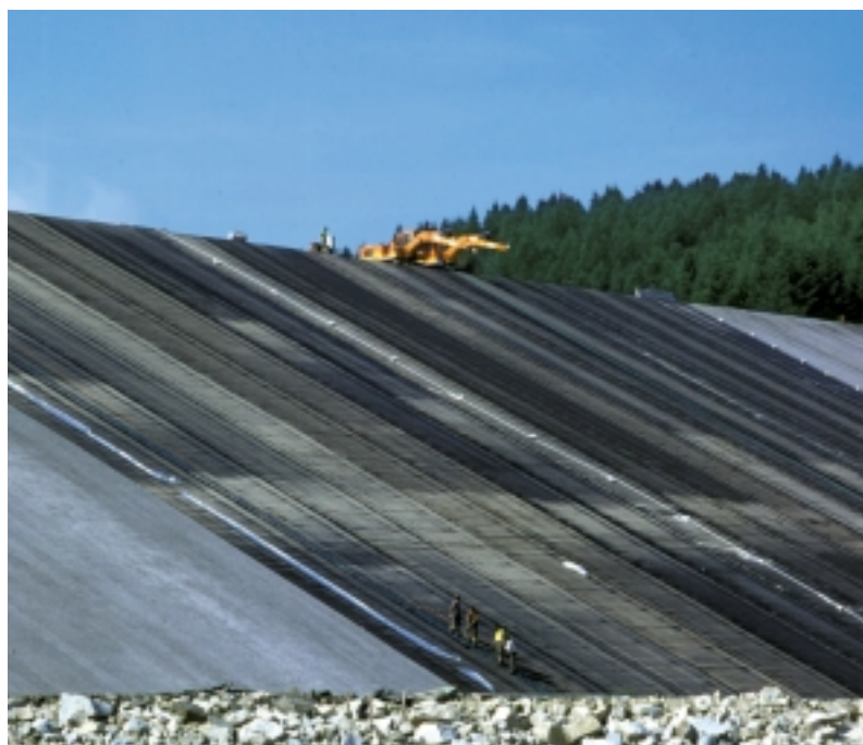
Colétanche upstream waterproofing membrane of Galaube dam (France).
