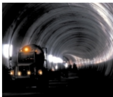
Losinger builds tunnels in Switzerland.
