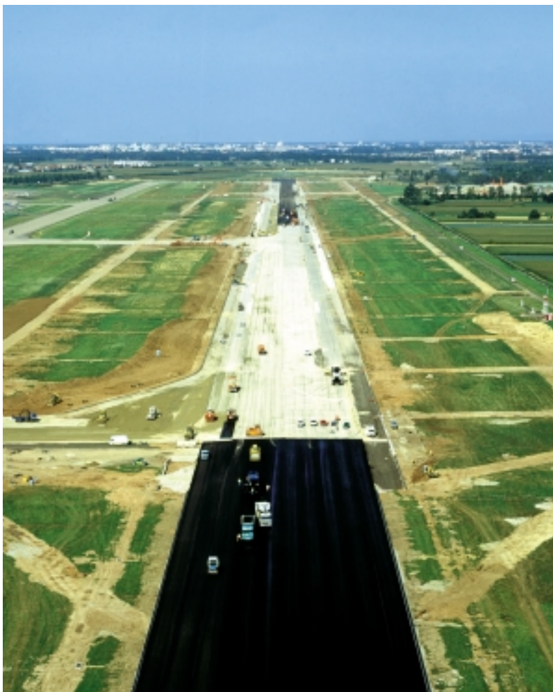
Renovation of runway at Strasbourg's Entzheim airport (France).
