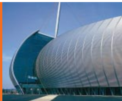
The Zenith arena in Rouen, built by Quille.
