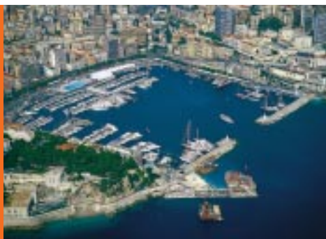
Extension works on the Monaco port.
