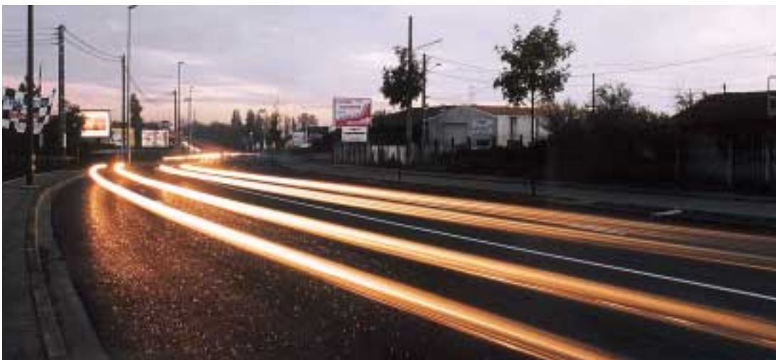
Scintiflex incorporates glass waste and combines visual and safety effects at night
