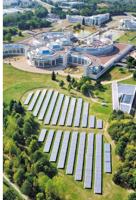
Challenger, Bouygues Construction's headquarters and a showcase for its expertise
