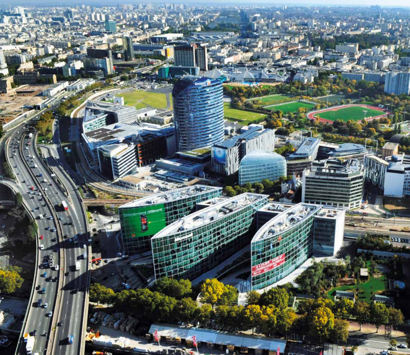
Managed by Bouygues Immobilier, IssyGrid® is France's first operational district smart grid, at Issy-les-Moulineaux, near Paris
