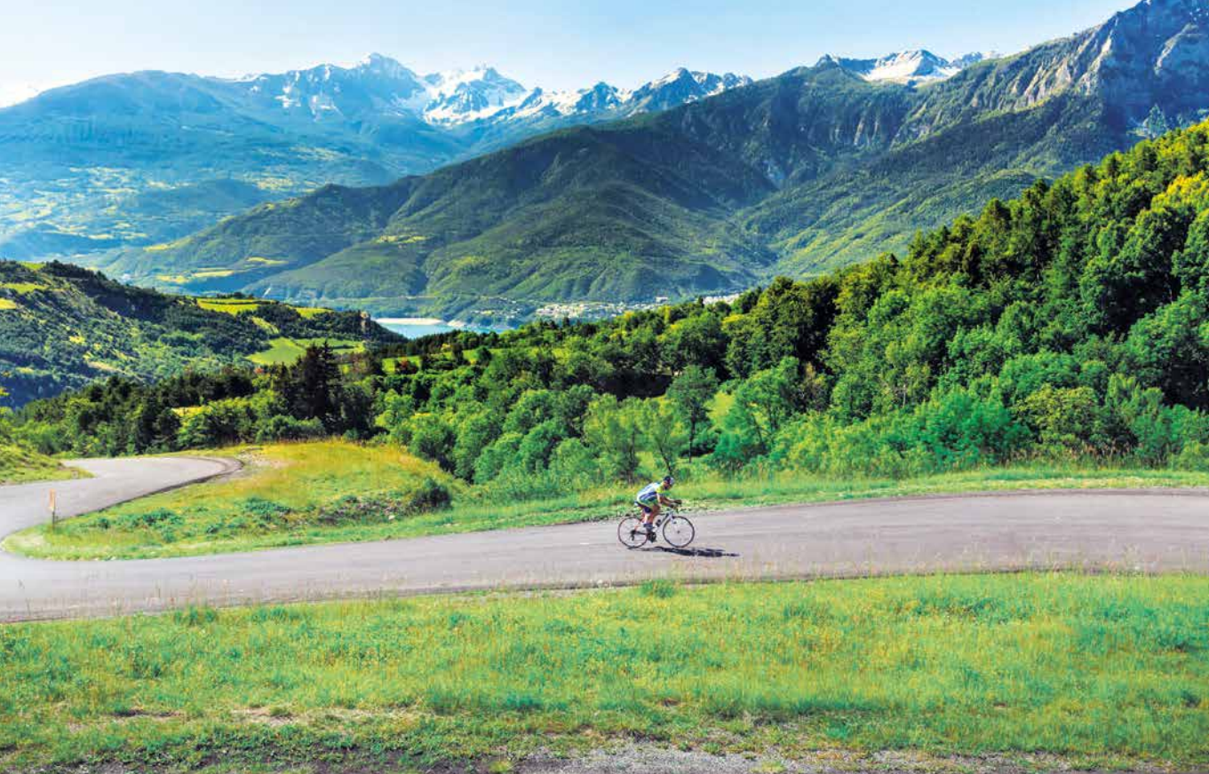
A section of the road between Embrun and Chorges in the French Alps resurfaced by Colas entirely with reclaimed asphalt pavement
