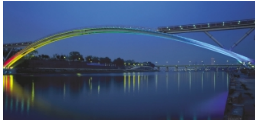
The Footbridge for Peace in South Korea. Ductal, a new concrete, made it possible to considerably reduce the thickness of elements and hence the quantity of raw materials used
