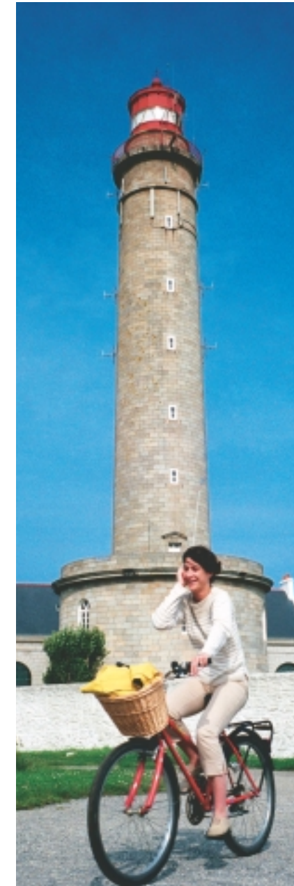
Bouygues Telecom preserves the regional heritage when installing its aerials
