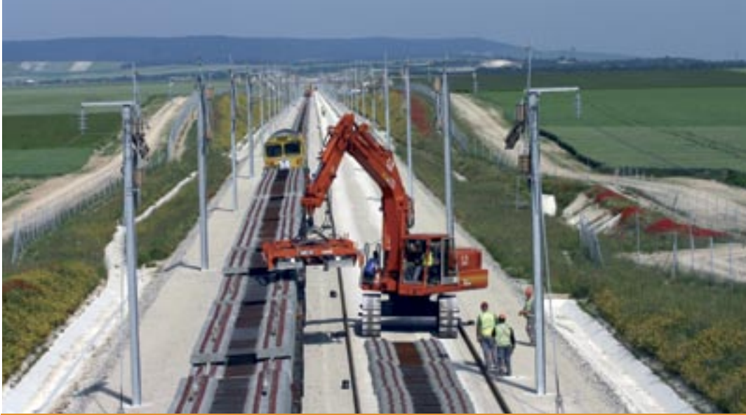
Tracklaying for the East European high-speed rail line
