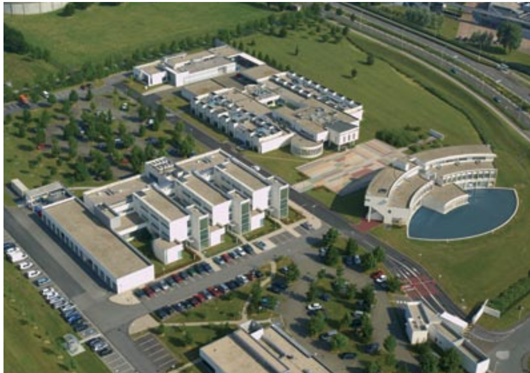
Campus for Science and Techniques in Magny-les-Hameaux outside Paris
