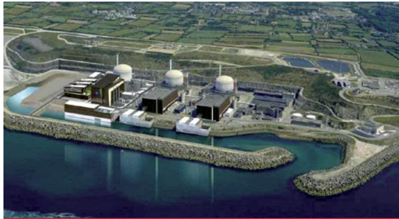
Bouygues and Alstom won the contract for the Flamanville nuclear power plant (France)
