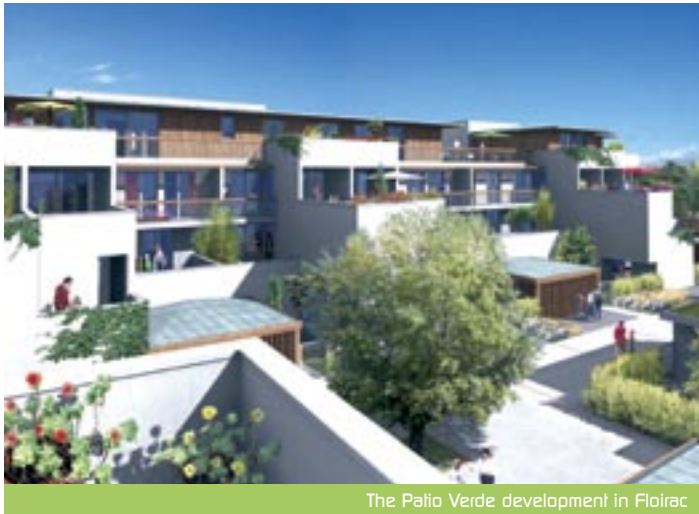
The Patio Verde development in Floirac
