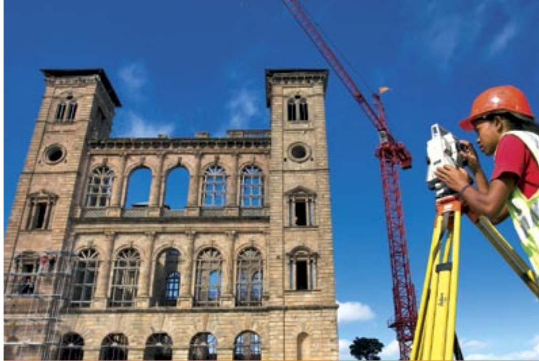
Rebuilding the Rova Palace in Madagascar under the aegis of UNESCO
