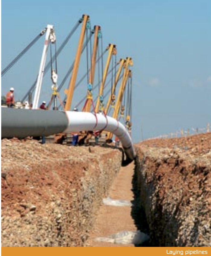
Laying pipelines
