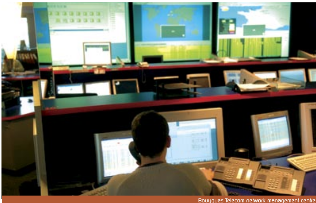
Bouygues Telecom network management centre
