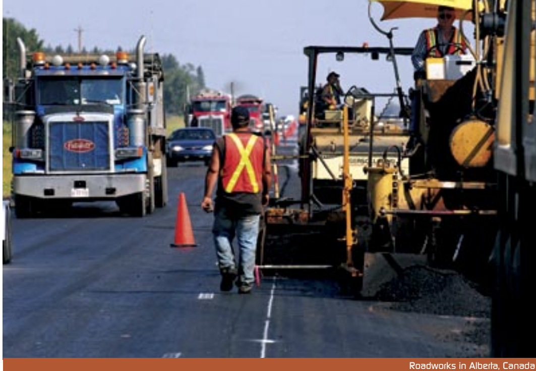
Roadworks in Alberta, Canada
