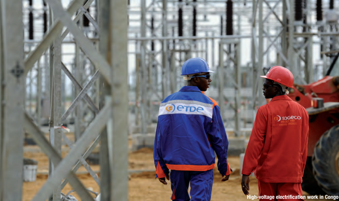
High-voltage electrification work in Congo
