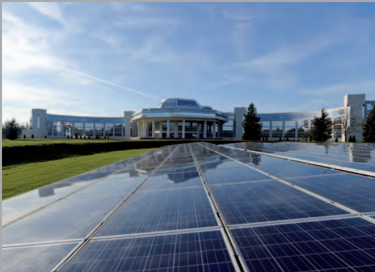
Challenger, headquarters of Bouygues Construction, undergoing environmental renovation
