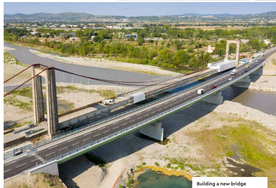
Building a new bridge (Manosque, southern France)
