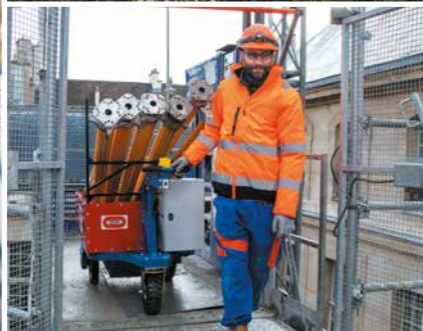
Kross Chantier, the smart trailer developed by Bouygues Construction in partnership with K-Ryole (a start-up) to reduce the level of arduous work for site workers
