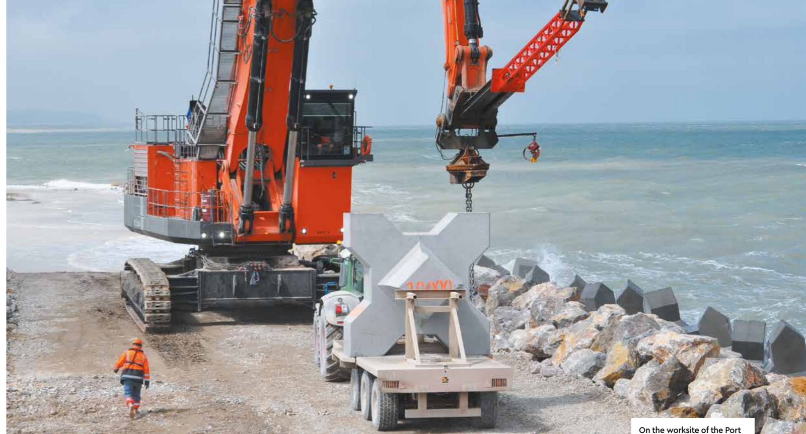
On the worksite of the Port of Calais extension project
