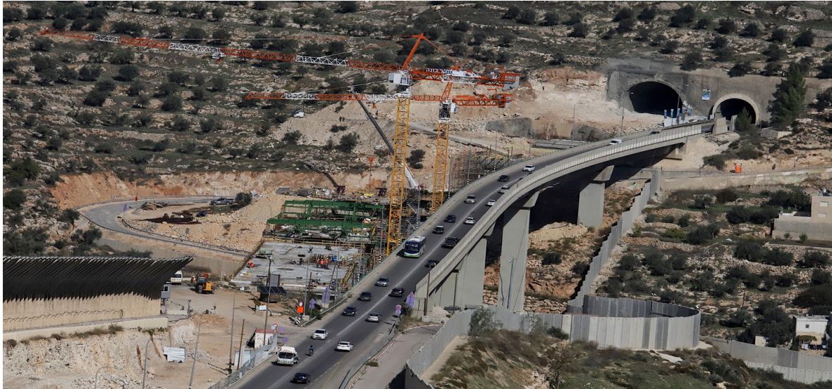
Construction to double the width of the Bethlehem Bypass Road (Highway 60 / the Tunnels Road)
