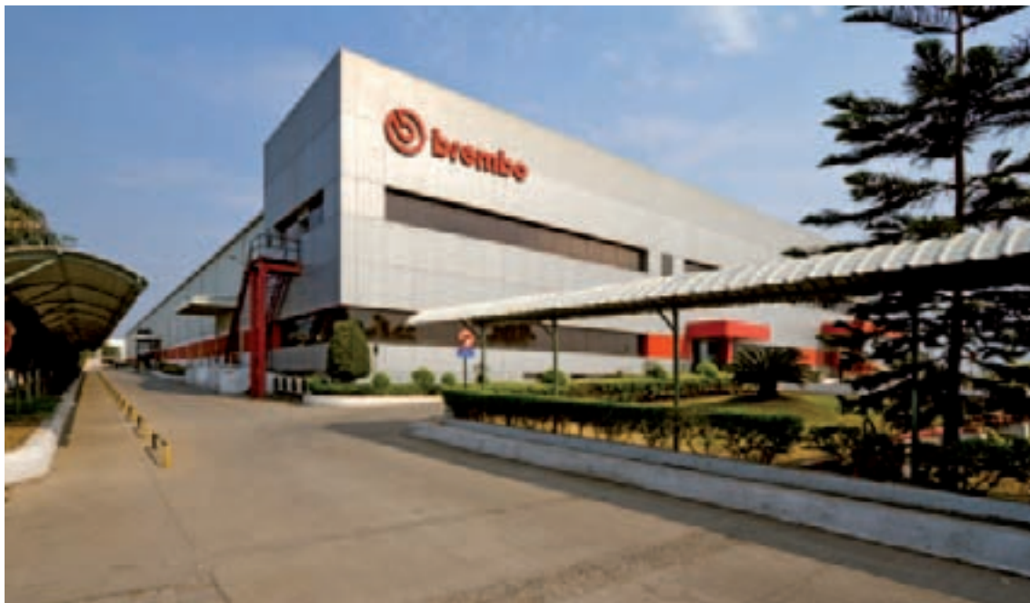
Pune motorbike plant (India).
