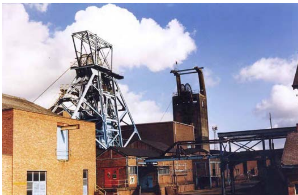
Figure 27 – Moorgreen Colliery (photograph courtesy of Anthony Kirby)
