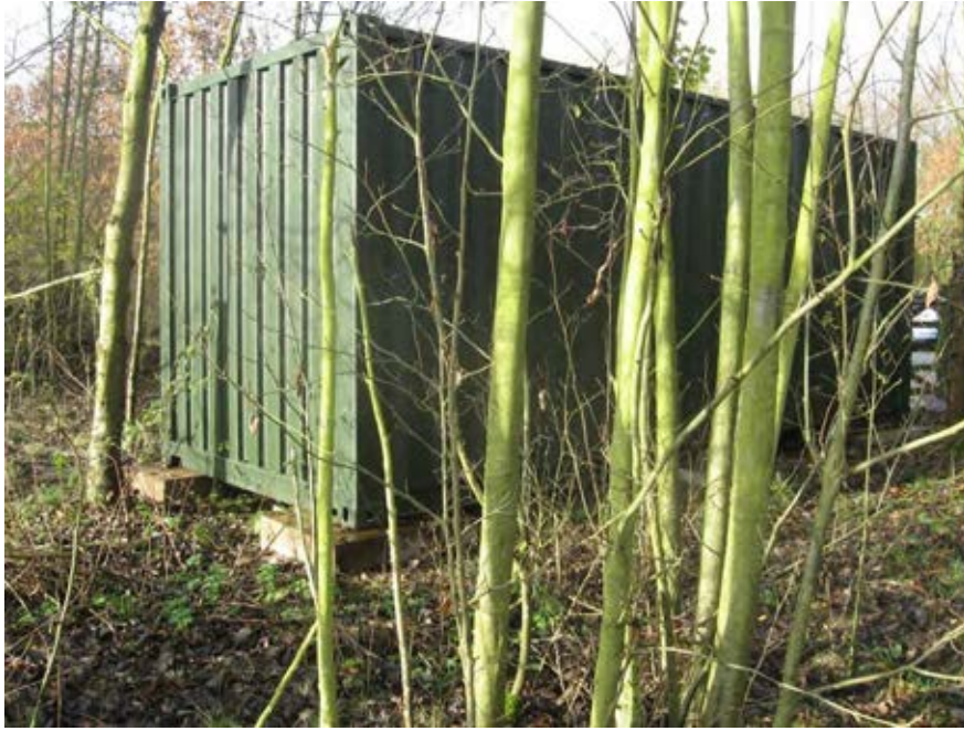
Figure 30 - Site Maintenance Store
