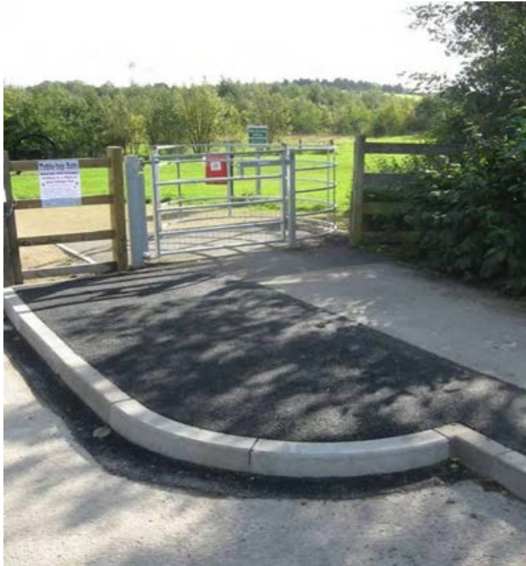
Figure 14 – Access gate for visitors with disabilities
