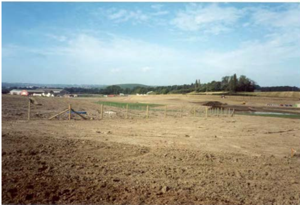
Figure 9 – Restoration Works September 1997
