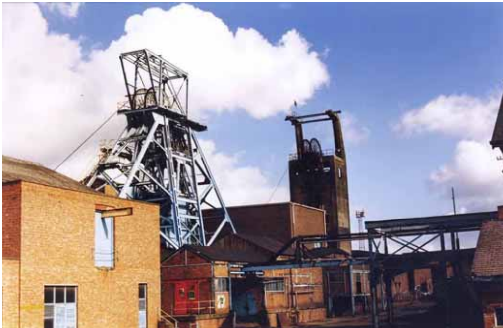
Figure 30 – Moorgreen Colliery (photograph courtesy of Anthony Kirby)
