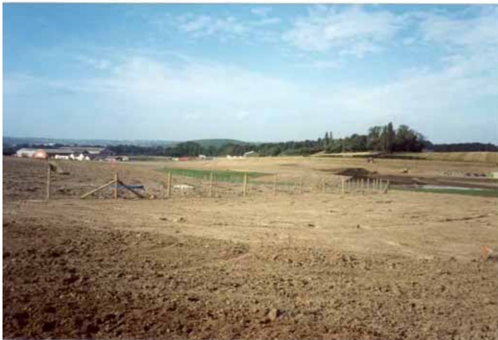
Figure 9 – Restoration Works September 1997
