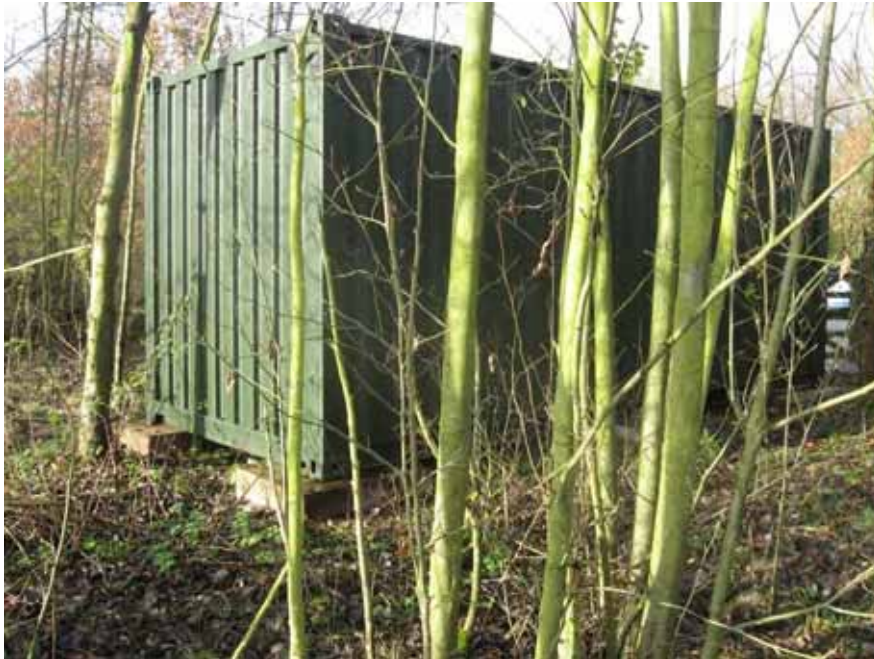
Figure 33 - Site Maintenance Store
