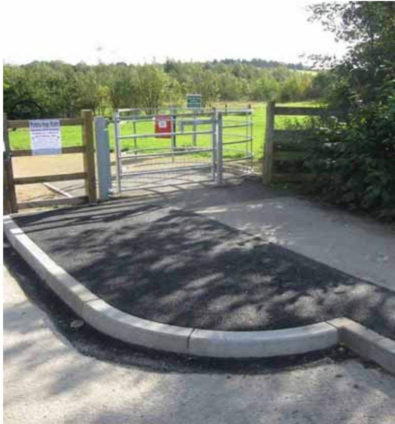
Figure 14 – Access gate for visitors with disabilities
