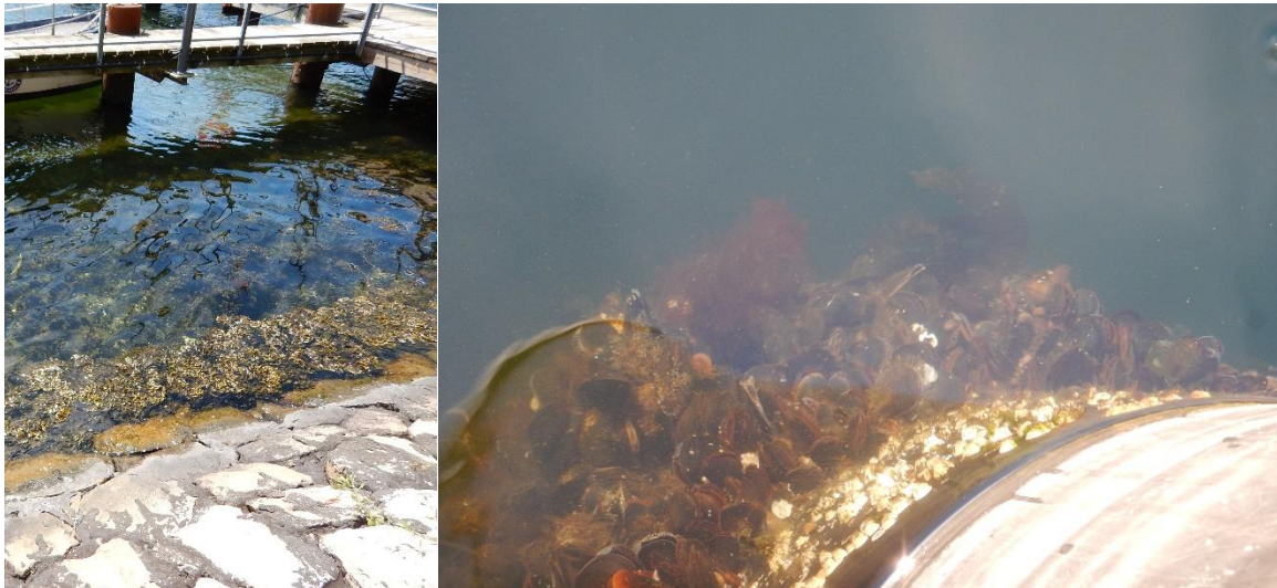
Figure 13: Rock filling with Fucus -cover (left) as well as fouling organisms on a pile mooring at the "Tiessenkai" harbor site in the Port of Kiel. (Image source: IfAÖ).
