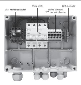
Fig. 2 - Electronic Control Drive
