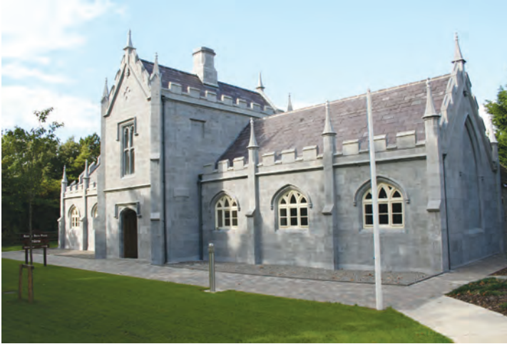
(fig. 129) ERASMUS SMITH BUILDING Church Street, Cahir (1818)
