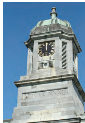
ST LUKE'S HOSPITAL
