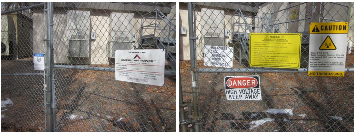
Figure 3: Signage Posted on Compound Gate
