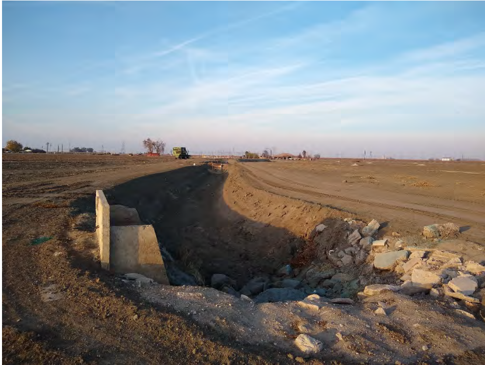
Photograph 4: Facing north along western boundary of the Project site (December 16, 2020).
