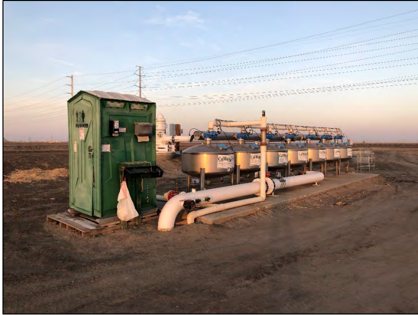
Figure 7: Media Filter Bank at Existing Reservoir
