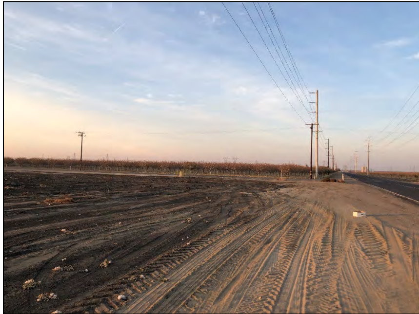
Figure 4: Buerkle Road and Wasco Way, facing North
