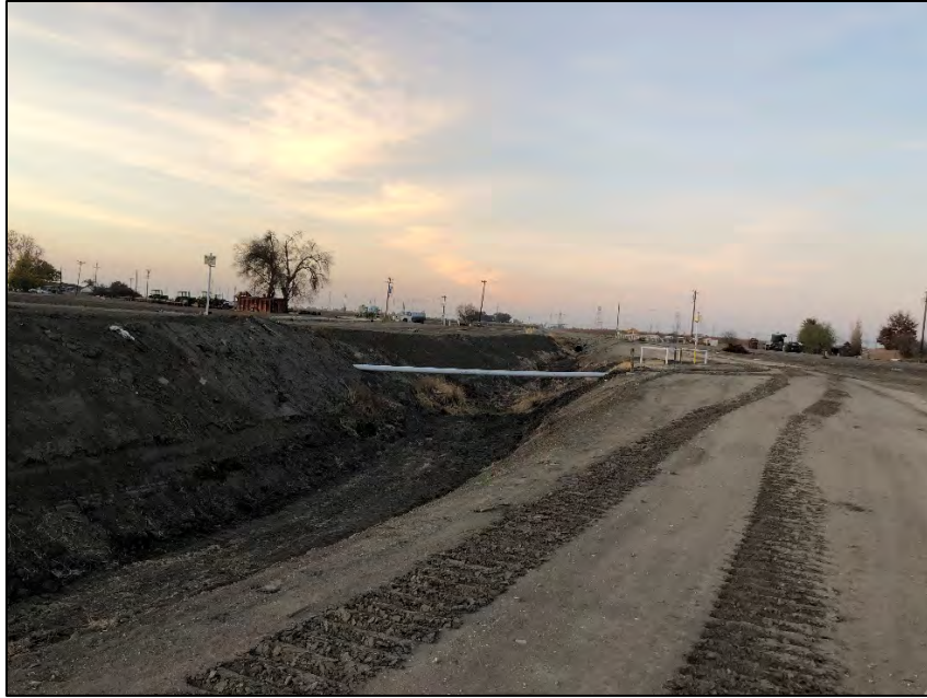
Figure 19: Main Drain Canal, facing North, with Gas Line Crossing
