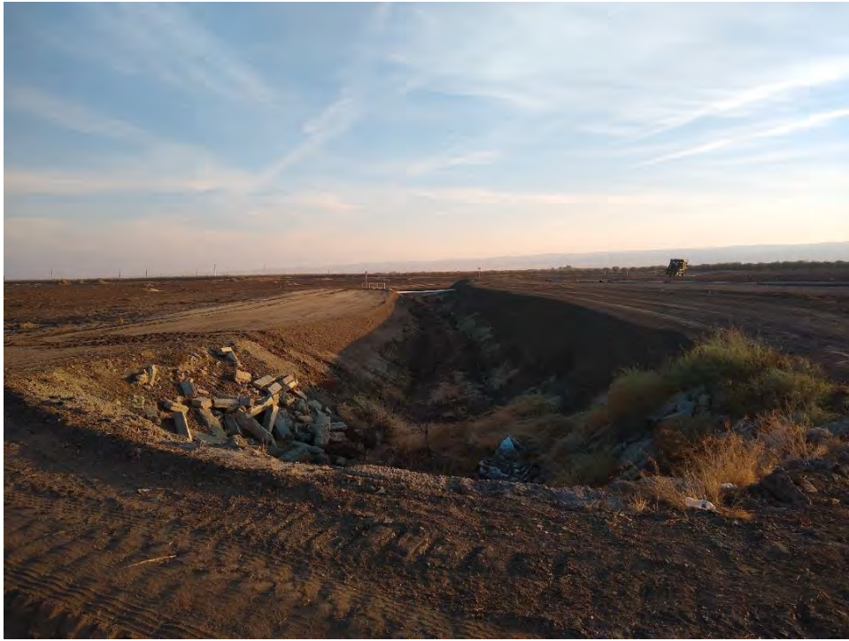
Facing south from northwest corner of the project site (December 16, 2020).
