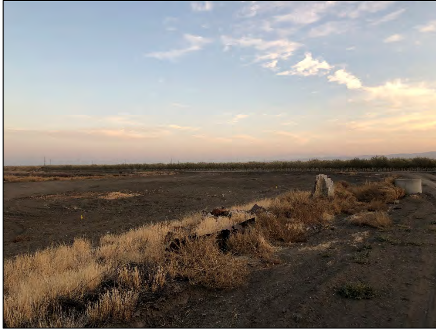
Figure 14: Main Drain Canal (Left) at Southwest Corner, facing Southeast
