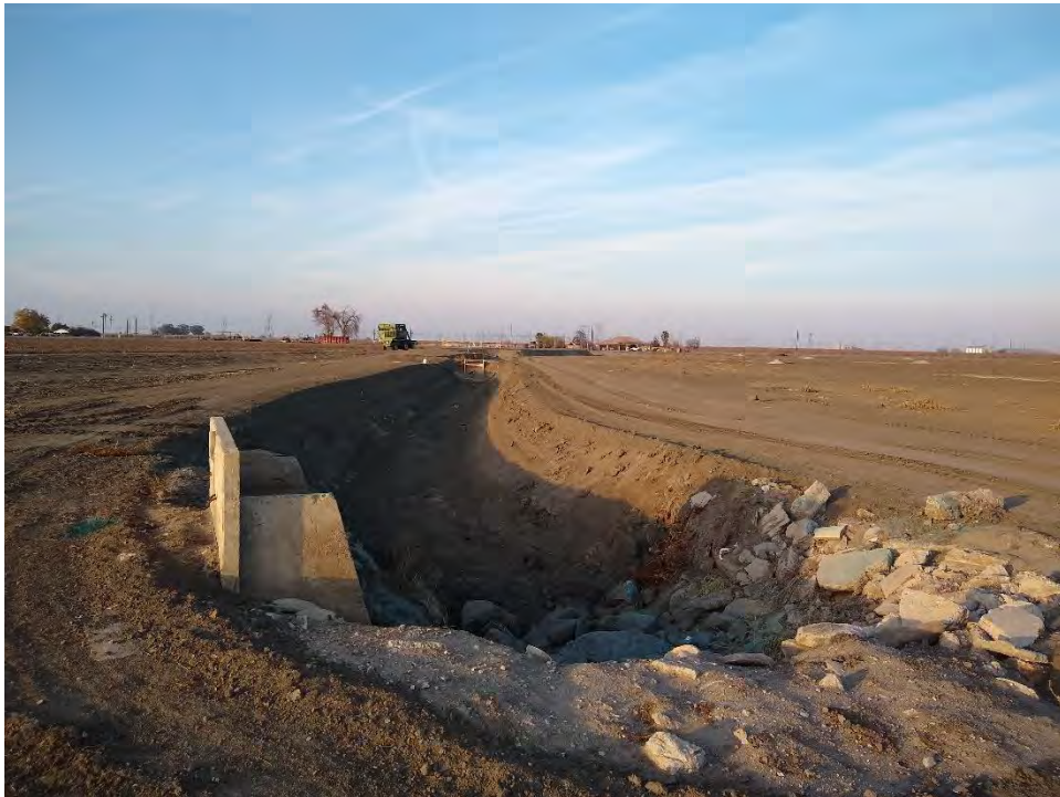
Facing north along western boundary of the project site (December 16, 2020).
