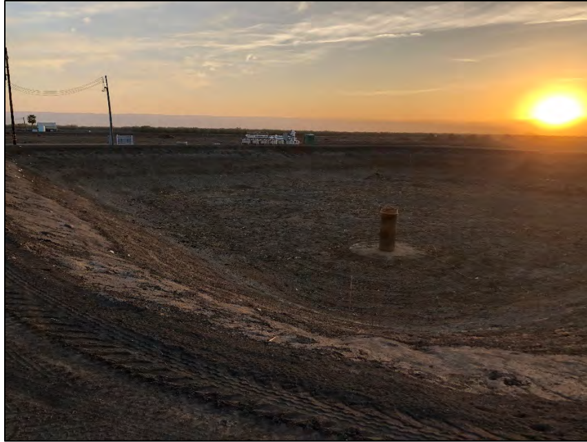
Figure 5: Existing Reservoir, facing Southwest
