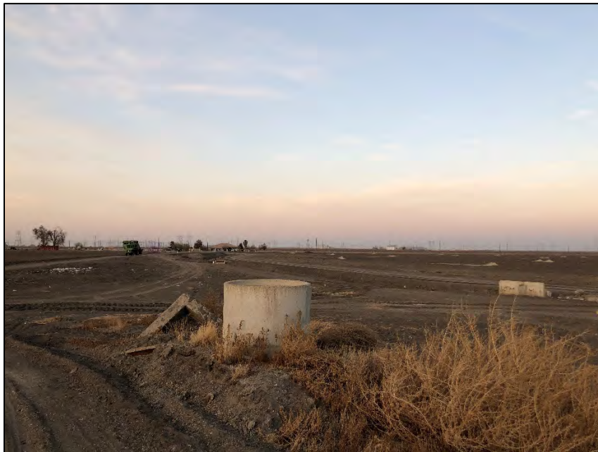
Figure 15: Turnout at Mirasol Ditch and Arizona Ditch, facing North
