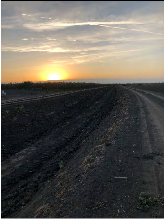
Figure 10: Arizona Ditch, facing West
