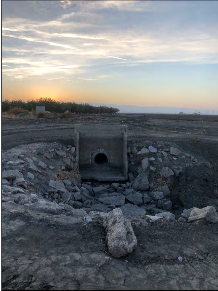
Figure 16: Concrete Outlet for Main Drain Canal to Arizona Ditch
