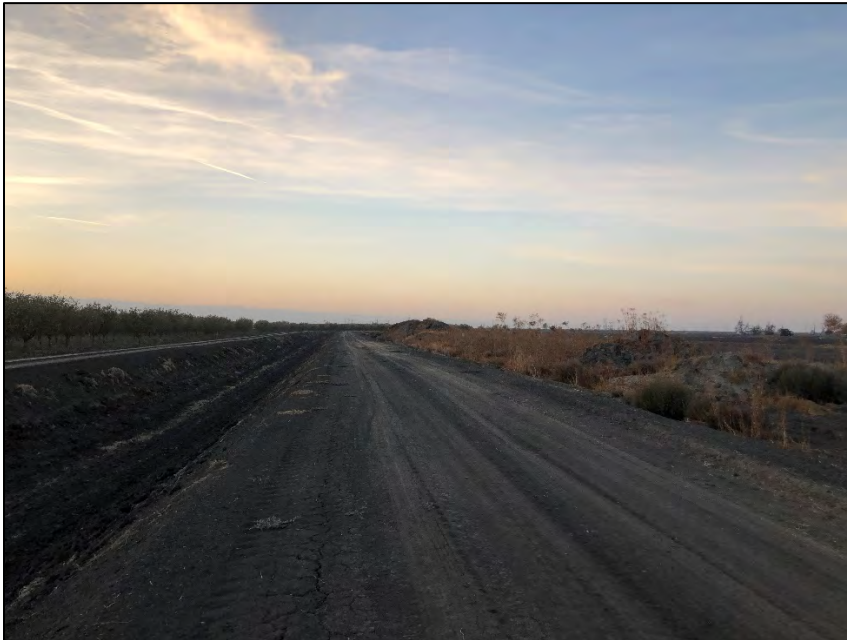
Figure 13: Arizona Ditch (Left) and Retention Basin (Right)
